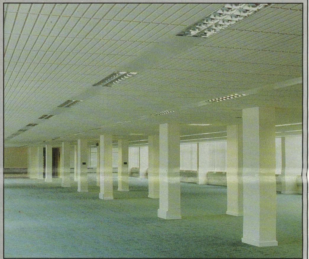
Five floors of the recently refurbished Tolworth Tower have been lit using recessed continuous Alterlux luminaires. Where a drop beam prohibited the use of recessed luminaires then surface continuous Alterlux was specified. Both products can be supplied with LG3 category 1, 2 or 3 louvres.
