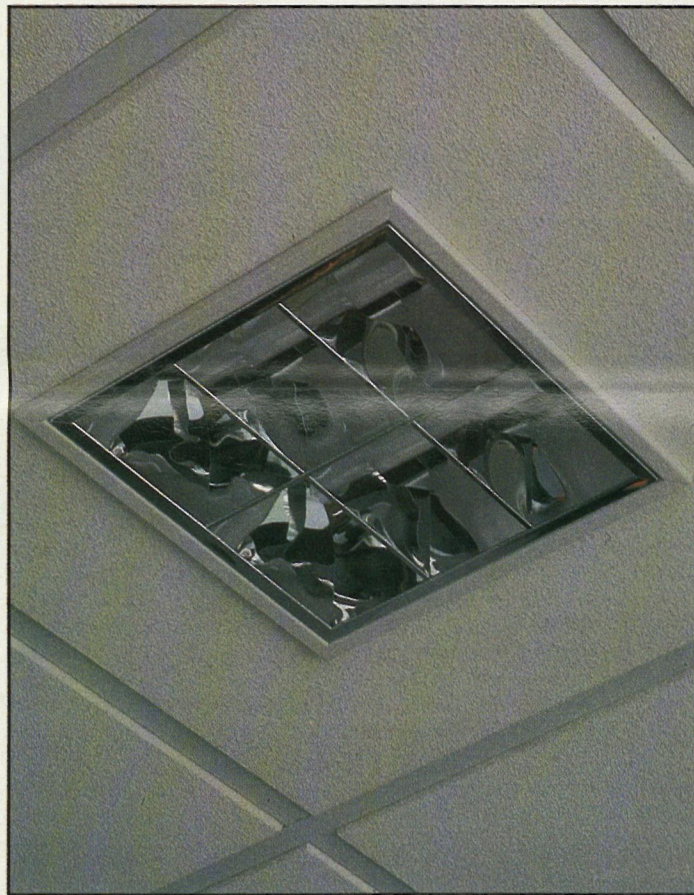
Five floors of the recently refurbished Tolworth Tower have been lit using recessed continuous Alterlux luminaires. Where a drop beam prohibited the use of recessed luminaires then surface continuous Alterlux was specified. Both products can be supplied with LG3 category 1, 2 or 3 louvres.
