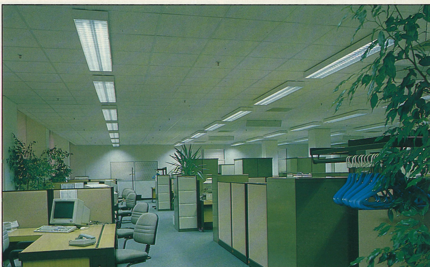
Siemens Module 3 surface mounted luminaires with Category 3 reflectors for general visual display work.
